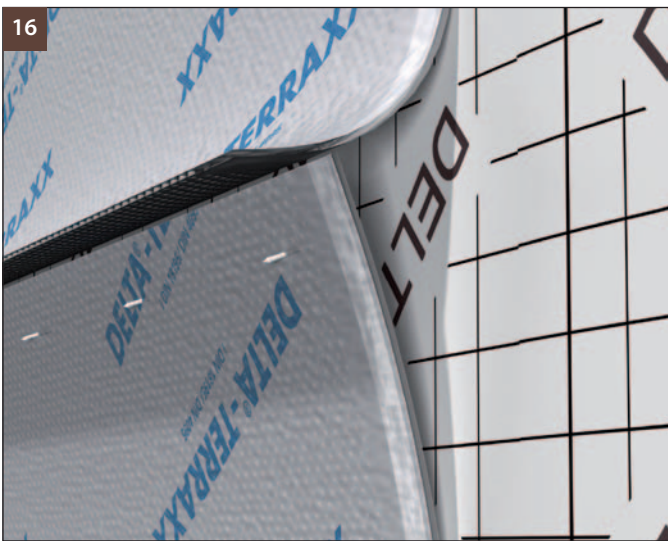
(Fig. 16) To extend a vertically installed sheet, insert another sheet at least 20 cm deep under its end.
