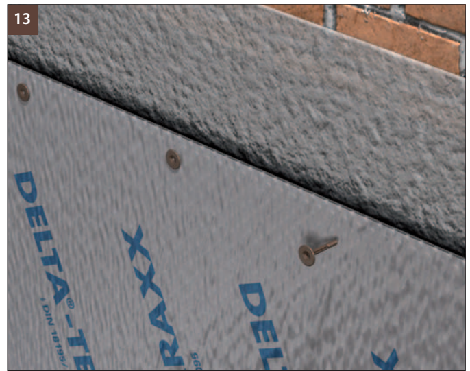
(Fig. 13) If the grade line is known, the sheet may be fastened immediately using DELTA®-MS DÜBEL.
