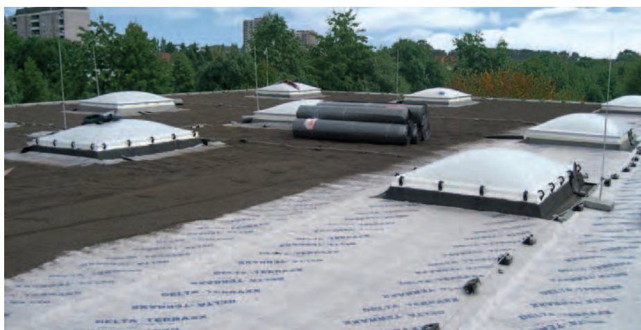
Laying is easy and cost-efficient.
