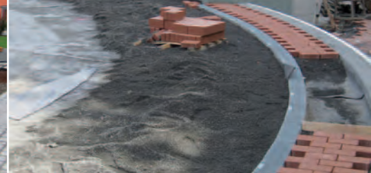
Sub-base being applied on top of DELTA-TERRAXX.
