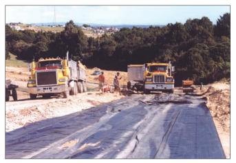
Woven geotextiles perform several important functions. Where separation is required on firm soils (CBR  $\ge$  8 %) a woven geotextile provides a strong and economical solution. The grades of geotextiles used for this are typically 100 to 250 gsm. For applications where a weak subgrade needs to be reinforced (CBR  $\le$  3 %) a high strength woven geotextile is used. These are classed by strength and are typically from 35 kN to 1000 kN.
