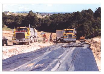
Woven geotextiles perform several important functions. Where separation is required on firm soils (CBR  $\geq$  8 %) a woven geotextile provides a strong and economical solution. The grades of geotextiles used for this are typically 100 to 250 gsm. For applications where a weak subgrade needs to be reinforced (CBR  $\leq$  3 %) a high strength woven geotextile is used. These are classed by strength and are typically from 35 kN to 1000 kN.
